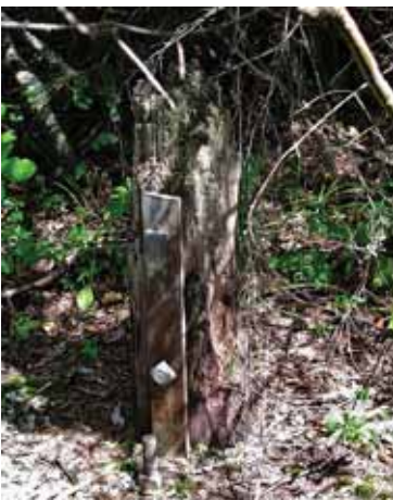
Bolts and steel anchored this telephone pole on the bare rock at Norway
