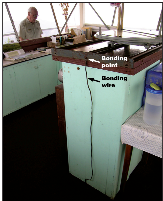
Figure 4—This bonding wire is attached to a fire finder inside a Forest Service lookout.
