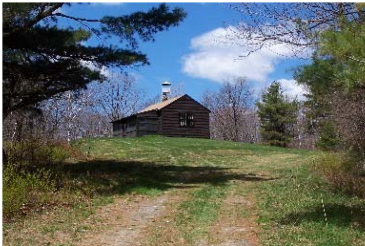
The Beebe Hill facility in May of 2007
