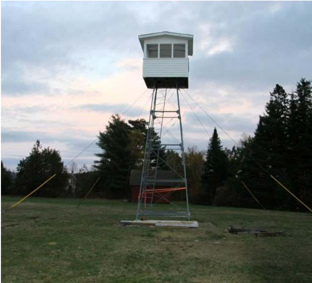
Norway Bluff – almost finished product; October 2012
