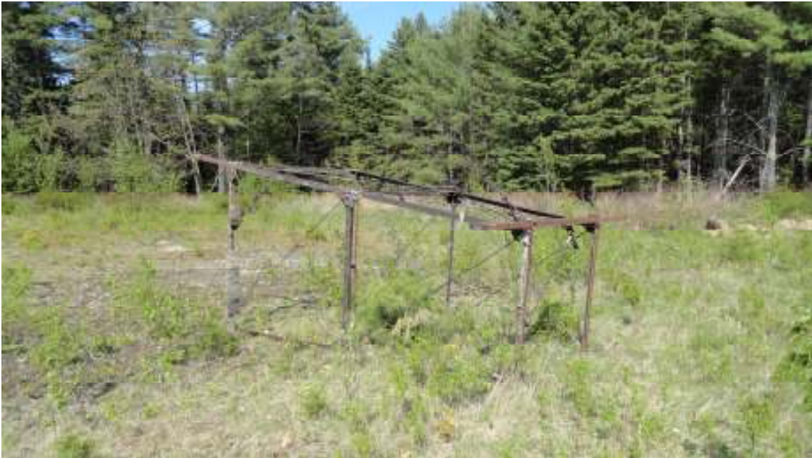
Big Moose Tower lays in a field next to the NREC facility on RT15 in Greenville
