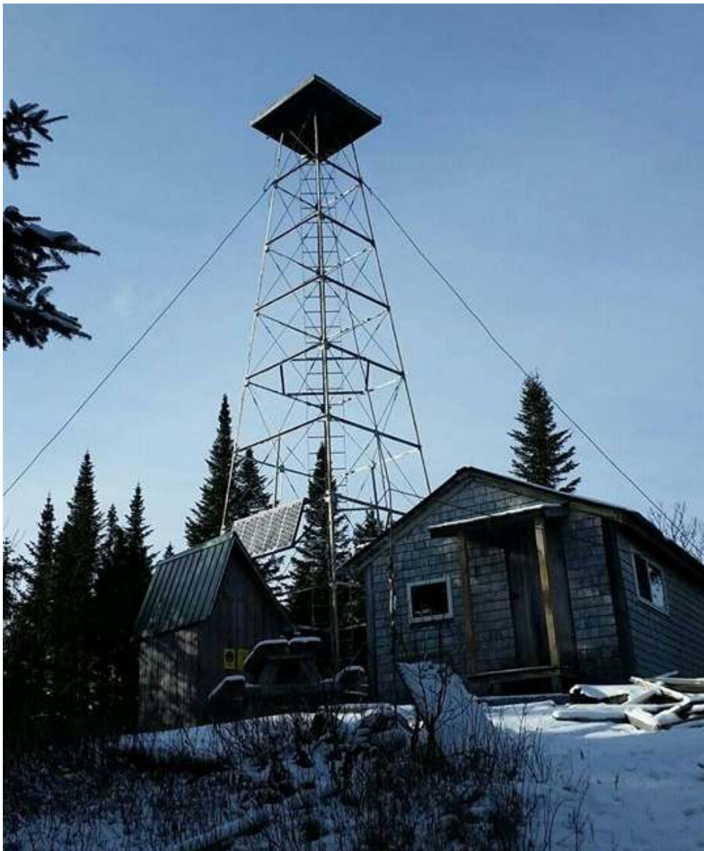
The cab-less Deboullie Mountain fire tower
