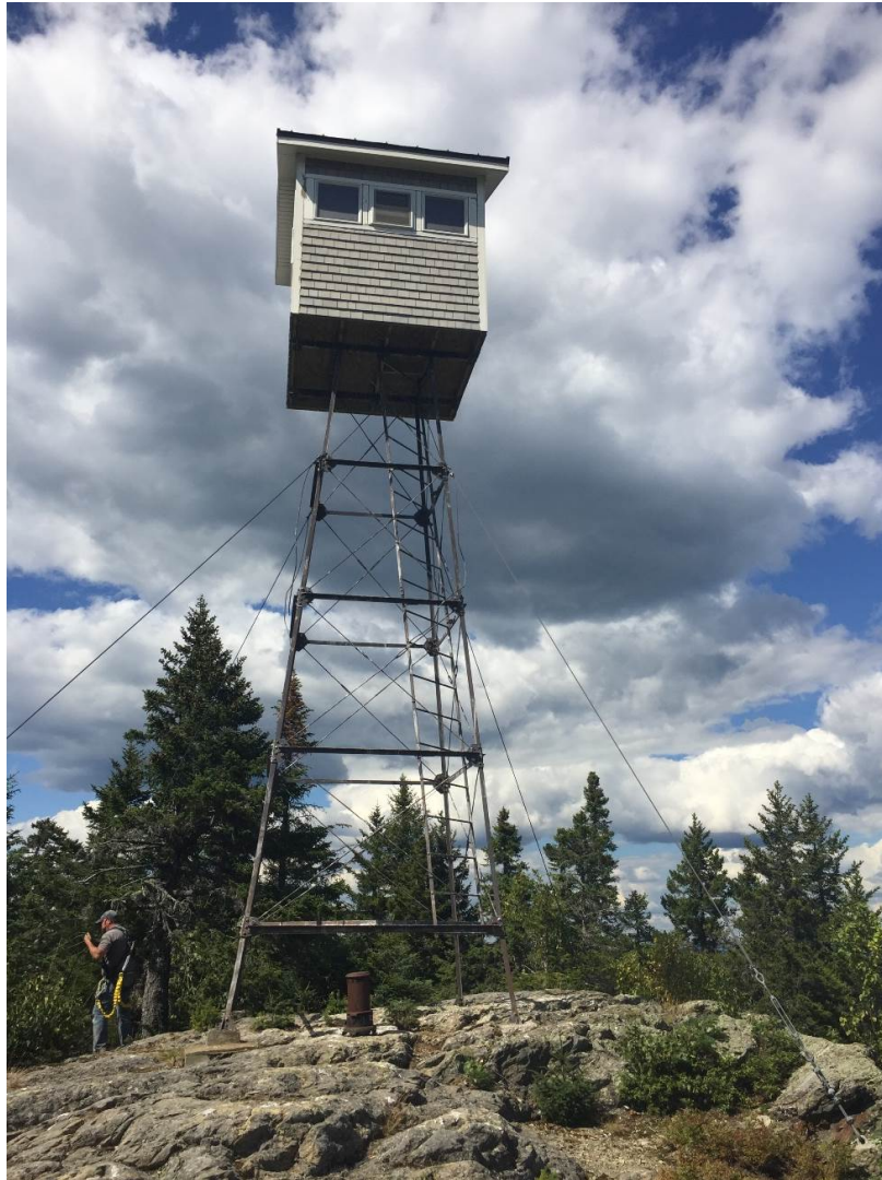
The new cab at Allagash Mountain fire tower
