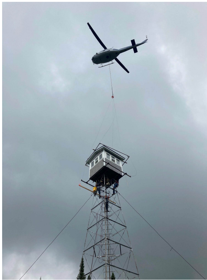
The new cab being installed at Deboullie Mountain fire tower
