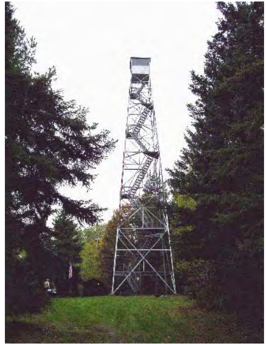
The Page Pond Hill fire tower International Derrick model 1933 - 76' 9" tall.
