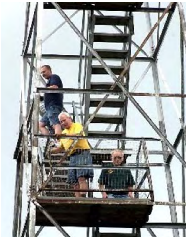
FFLA members Eric Hepperle, John Wheeler and deputy state director Bob Eckler install the wire safety meshing.
