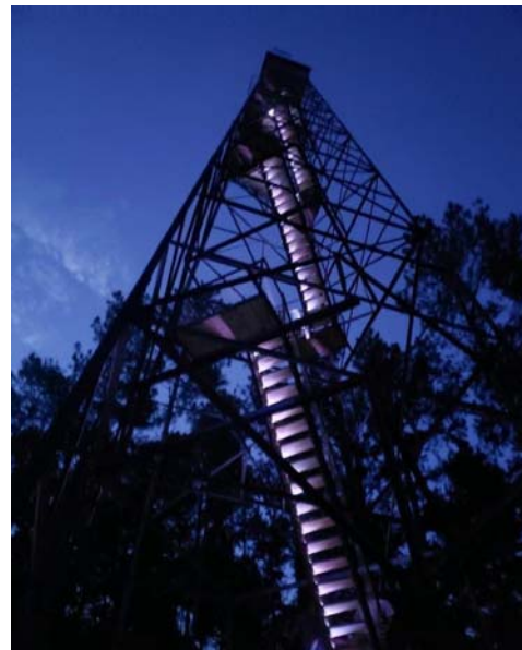
Tower with LED Lights on legs to light tower at night.
