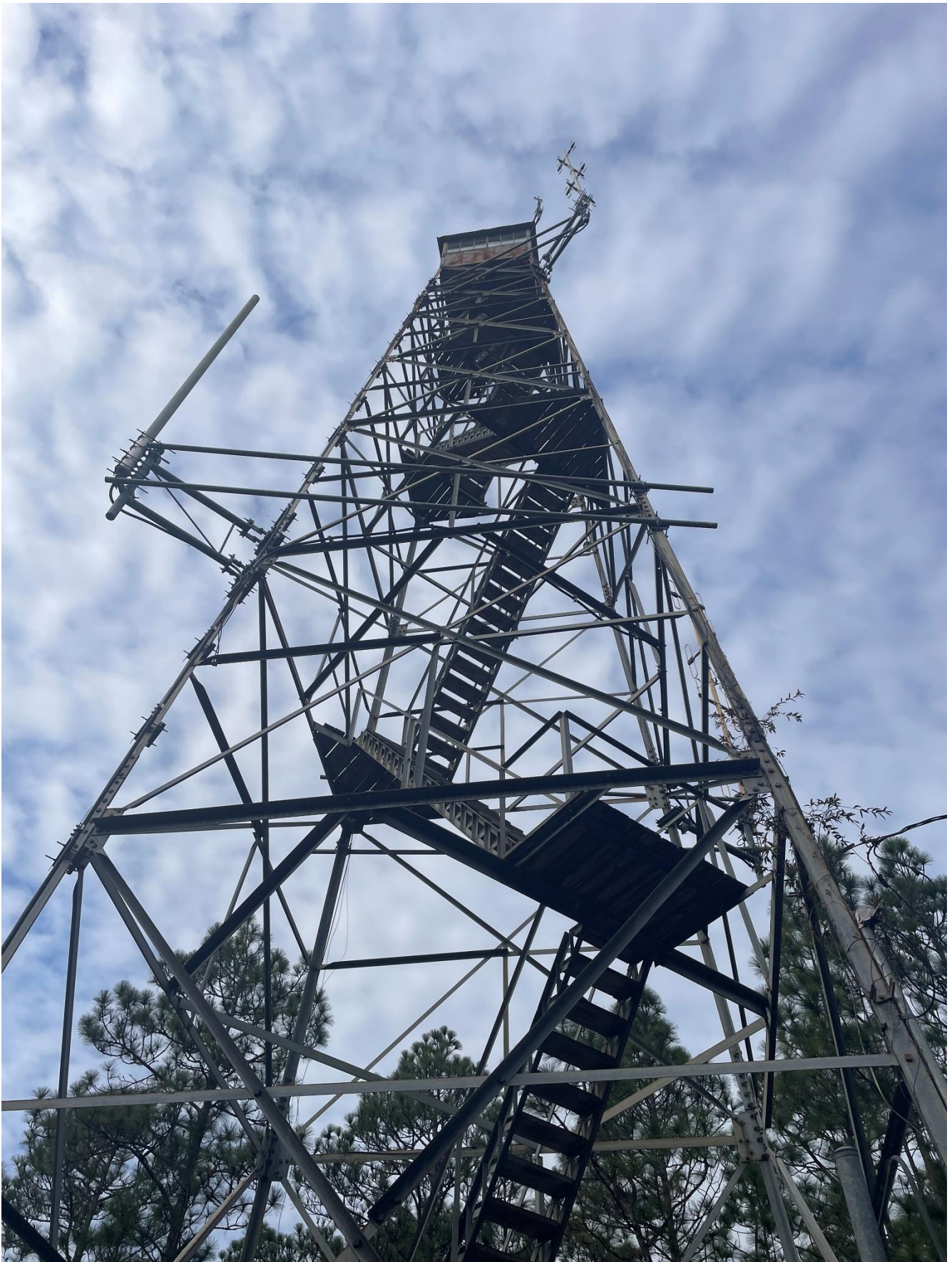
Figure 7. Rosemary Fire Tower, facing north and upwards.
