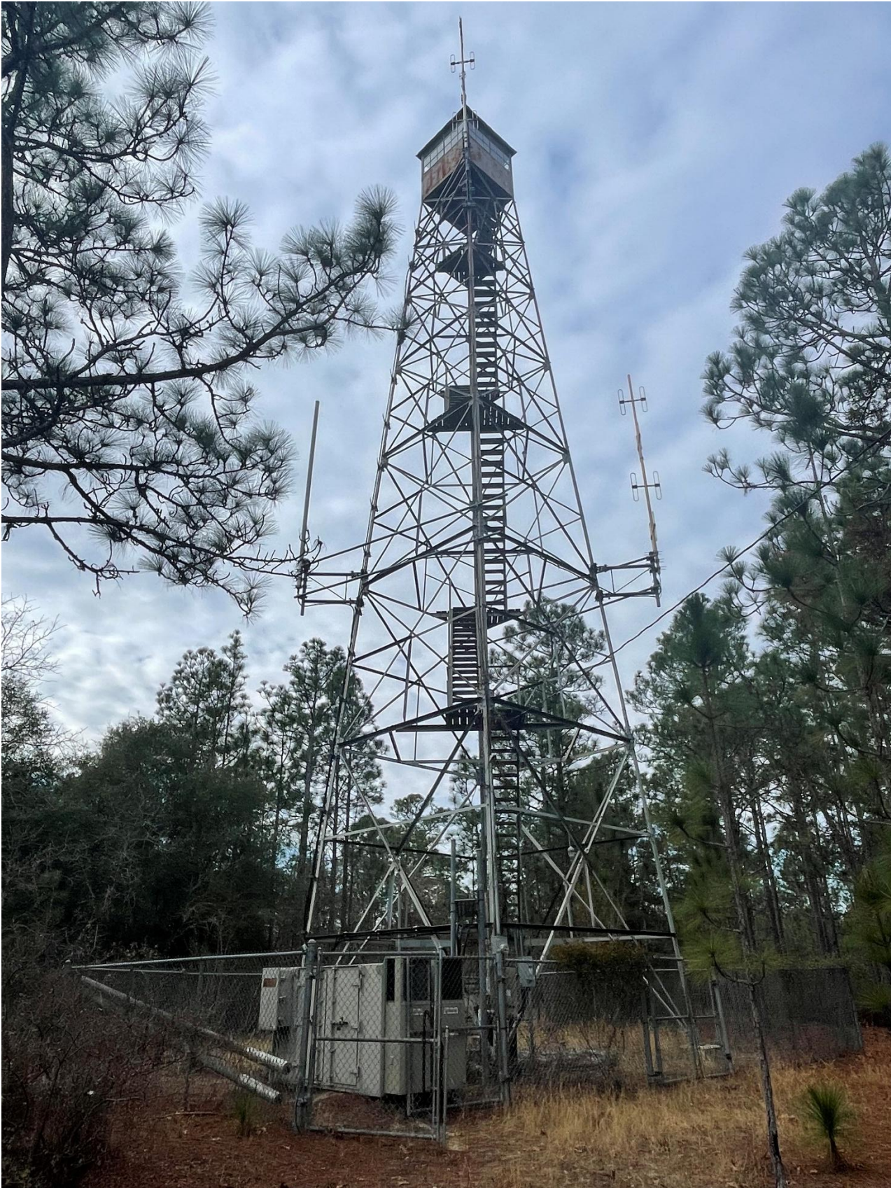
Figure 6. Rosemary Fire Tower, facing northwest.
